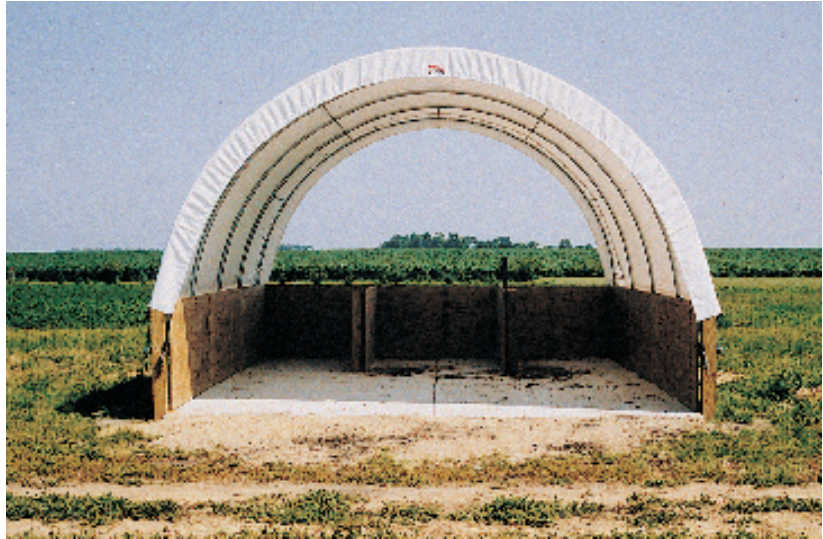
Hoop structure for composting with three bins.
