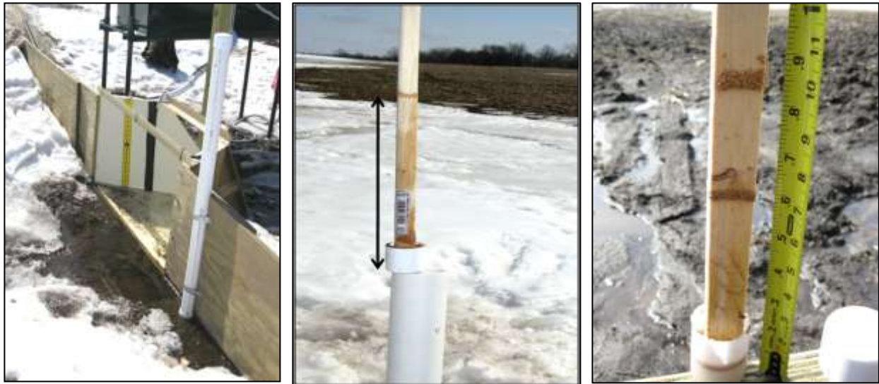
Figure 11. CSG location on upstream wingwall and cork measurements following a runoff event.
