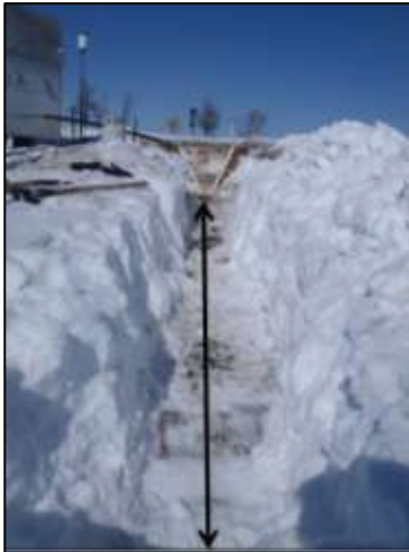
Figure 15. Snow removal area downstream from flume.
