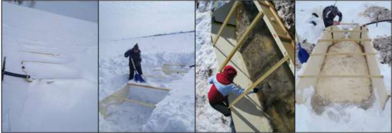
Figure 14. Progression of flume cleaning. 1) Shovel and remove excess snow. 2) Carefully melt and chip out any ice. 3) Clear upstream and downstream flow paths.
