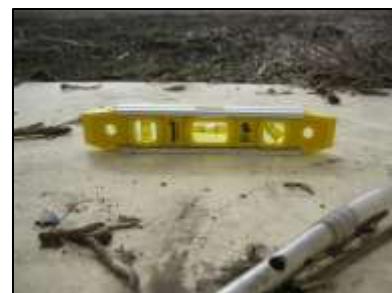
Figure 20. Checking flume levelness.
